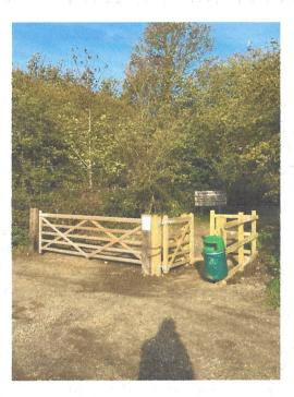
No latch has been provided for the pedestrian gate. The original litter bin has not been securely fixed in place. A large puddle forms in the pedestrian entrance way after heavy rain.
